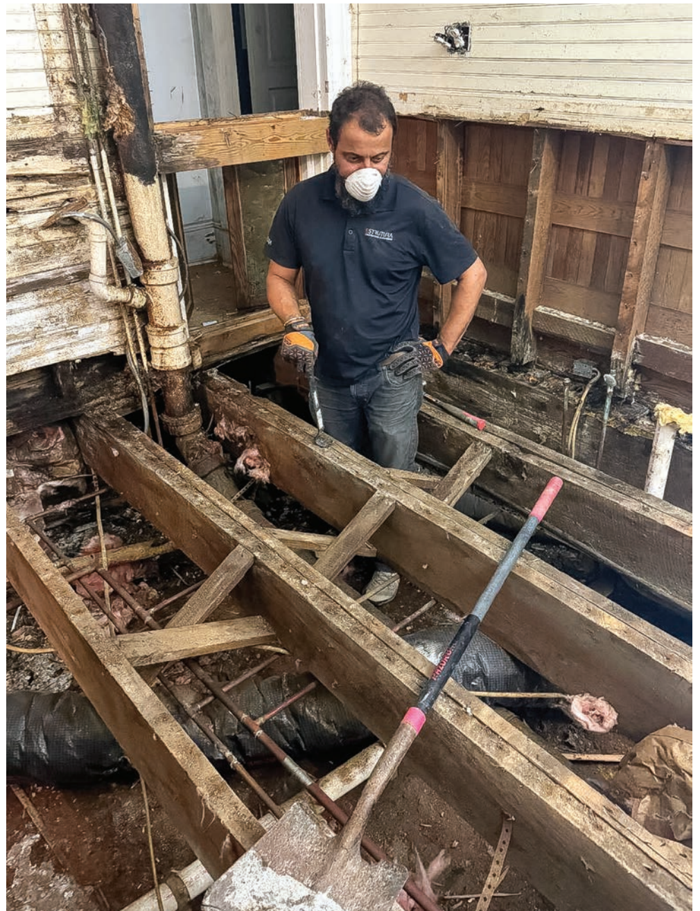
Ronny works on replacing the floor during the restoration process. (Submitted photo)
