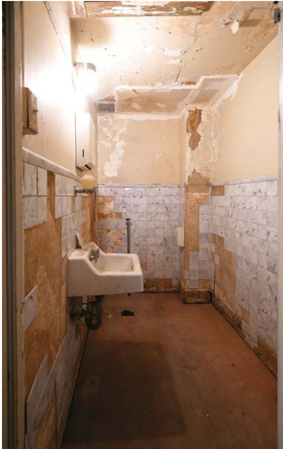
The remaining original bathroom in all its glory.
