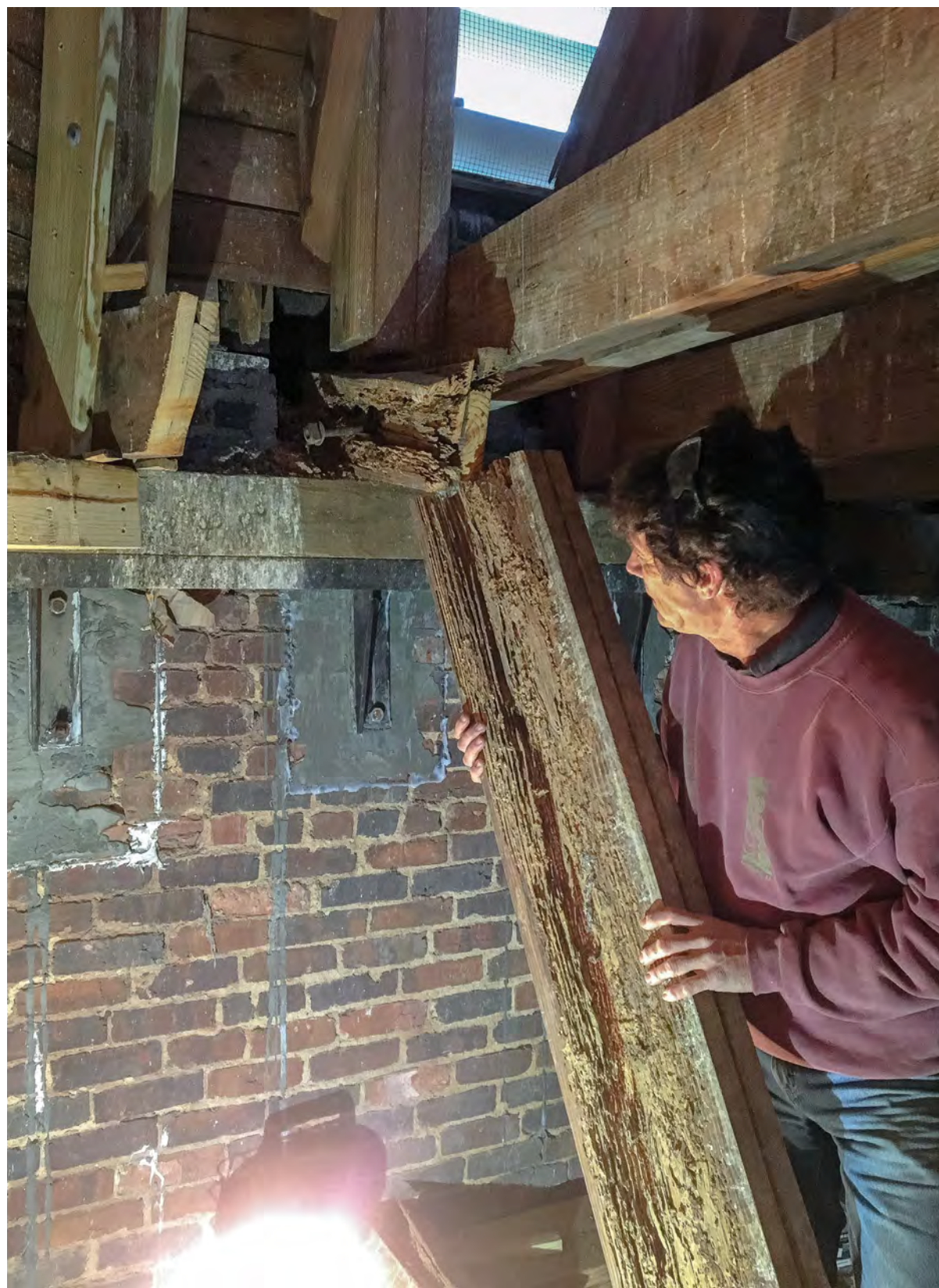
Al Wilson removes termite-damaged beams from the Bell Tower. (Photo courtesy Al Wilson)
