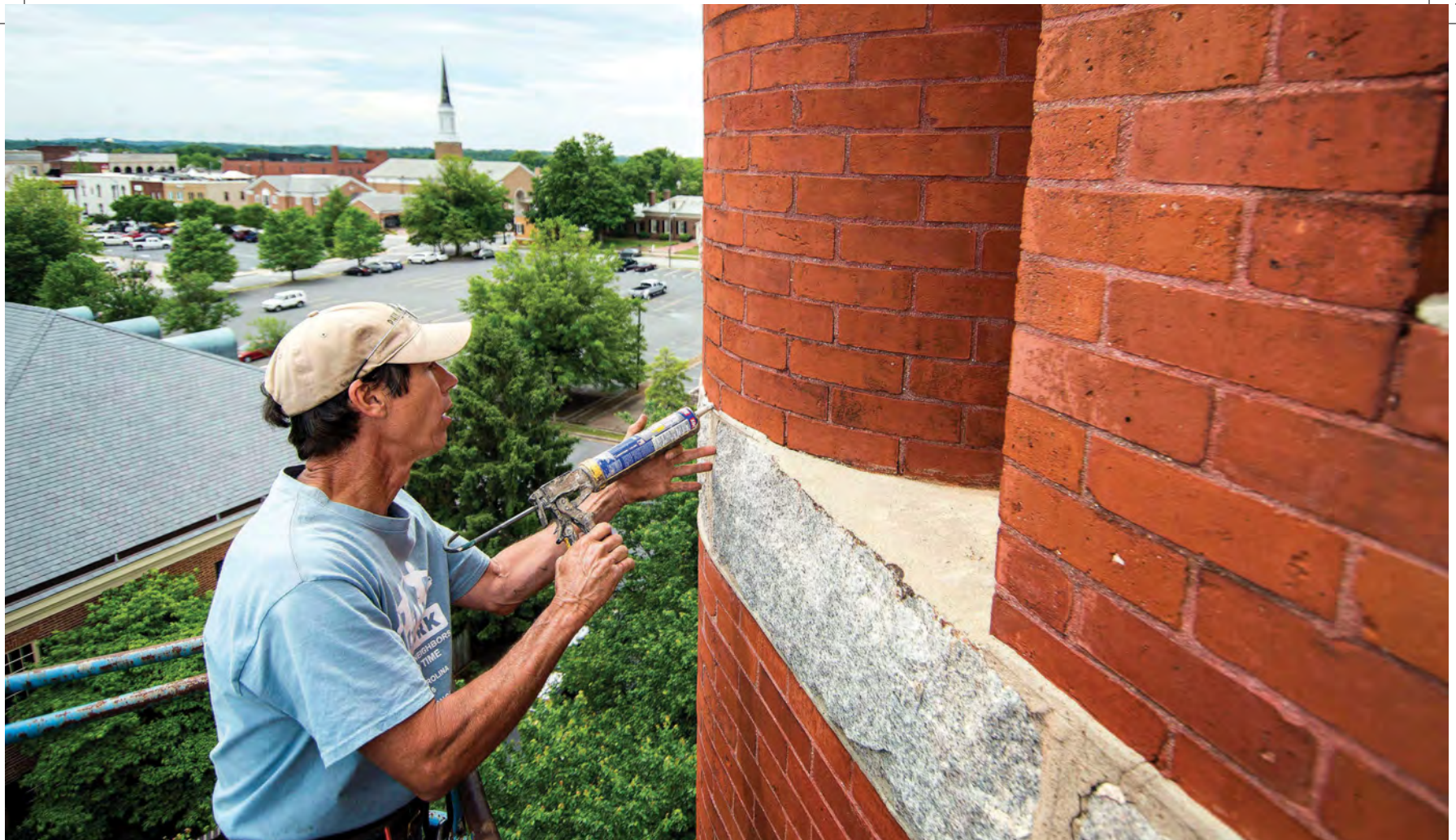
Al Wilson uses a 124-foot tall lift to place a bead of caulk on those hard-to-reach areas on the exterior of The Bell Tower in 2017. (Jon C. Lakey, Salisbury Post file photo)
