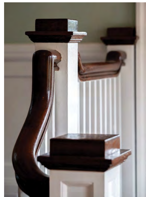
Below: The original stairwell survived many years of neglect.
