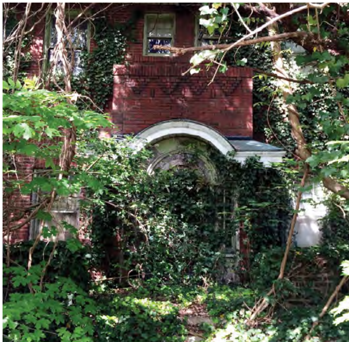
The 128 W. Thomas St. house before renovation. (Submitted photo)
