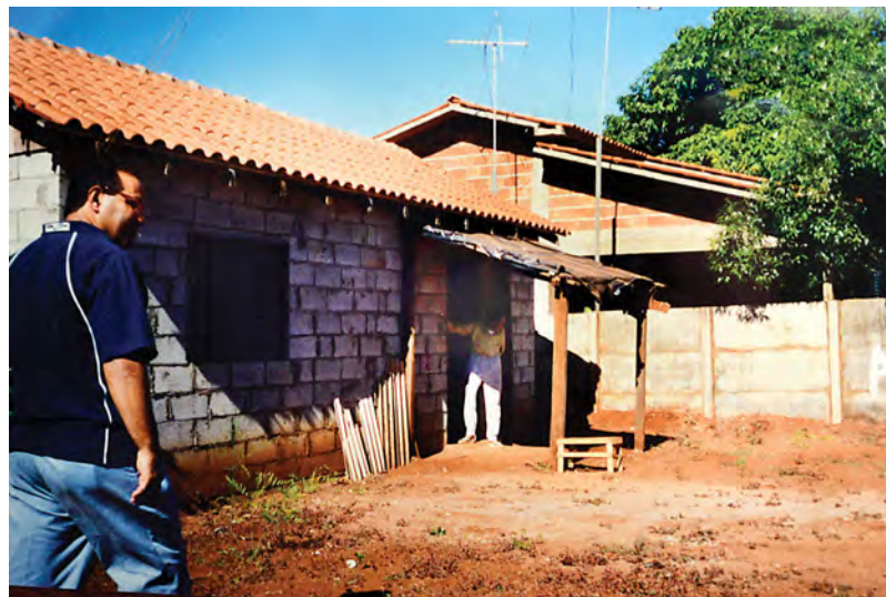
A Habitat house in Brazil in that Bob Harris helped build.
