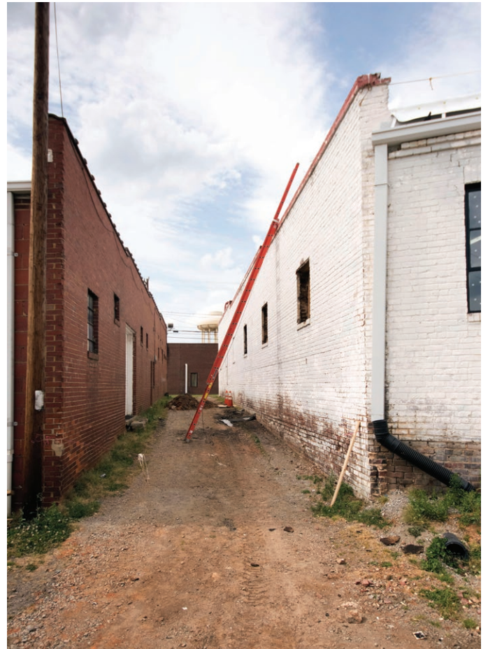
This alley will be closed off so that a grain silo can be placed next to the building to feed into Morgan Ridge’s new brewhouse.
