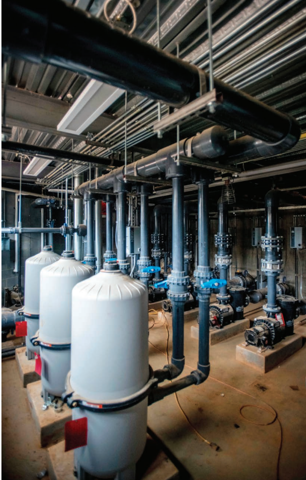
Clockwise from far left: Climbing equipment in the children's play area; construction crews work on the roof for the performance stage; the amount of piping and pumps required to move the water across the face of the wall; landscape architect and Rowan County native Allison Merriman worked on the project.
