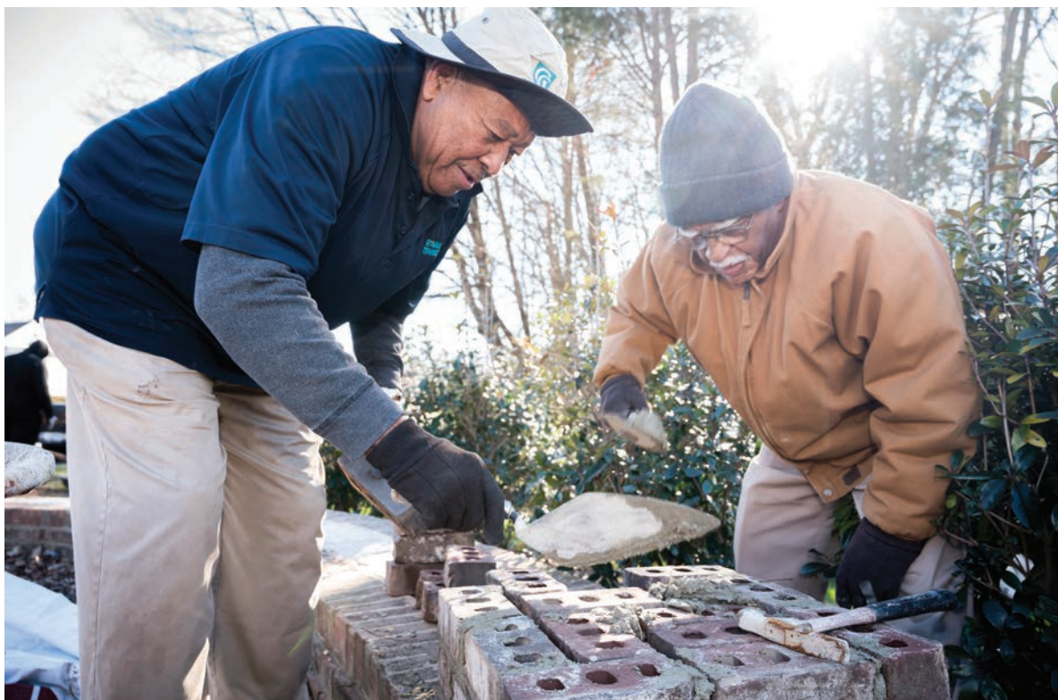
Above: Lovie Reid stands in front of the Livingstone College perimeter fence that he built.
