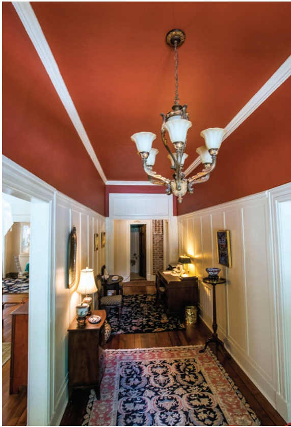
Above: To make up for crumbling plaster, the hallway chair rail was moved up.
