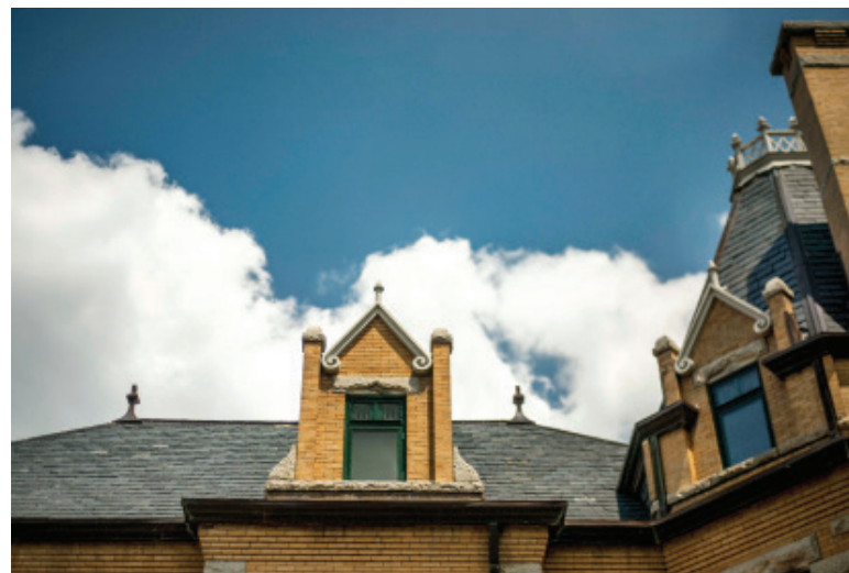
The house has a roof of Vermont slate.
