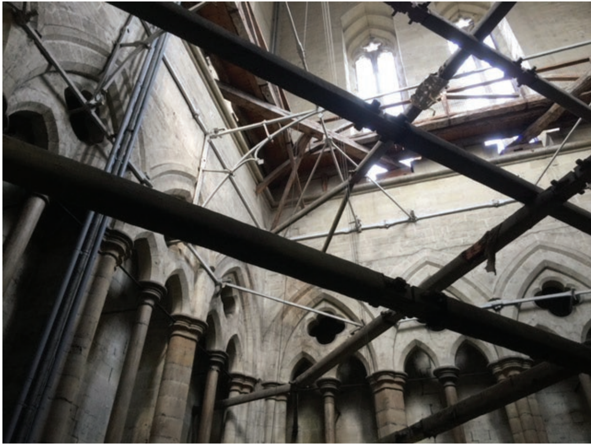
Above: Extensive bracing is needed throughout the Cathedral. Right: The ruins of the Old Sarum Cathedral.
